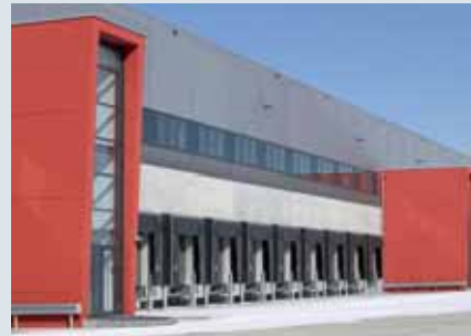
Immogate logistics centre, Munich
