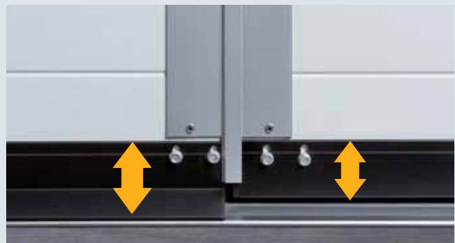
A separately adjustable bottom seal for both doors compensates for any slight unevenness in the floor.
